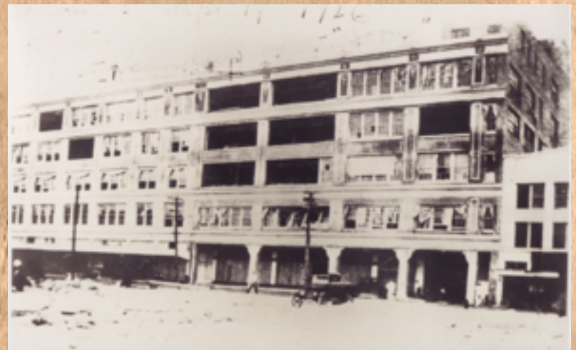
Windows blown out of a factory.
