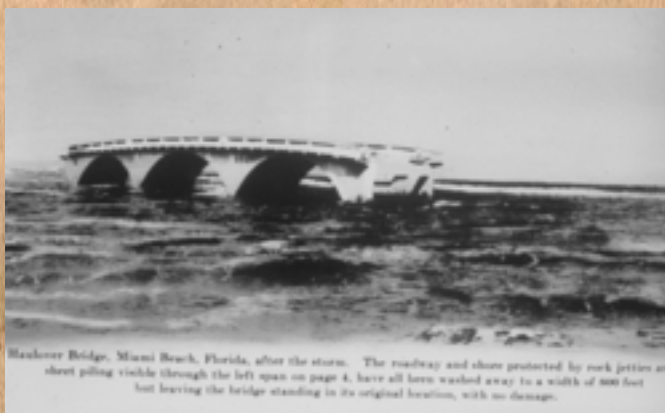
Before and after pictures of the Haulover Bridge, Miami Beach, Florida.
